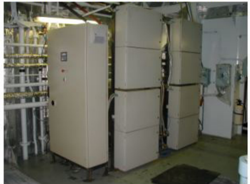
Above. OT-100 system delivering 4000g/hr ozone @ 2 bar for treatment of ballast water onboard MV Taronga.
